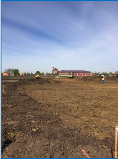
Bulldozers working together to clear the land.
