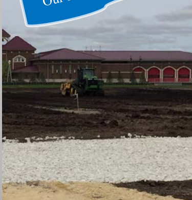
Yes, our building will be bigger and taller!
