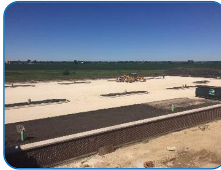
North Parking Lot Gravel
