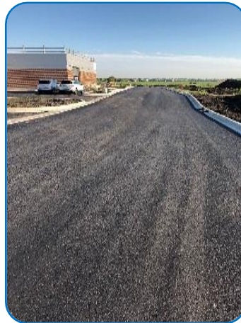
Binder Coat Paving
