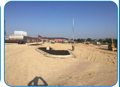
Parking Lot Preparation
