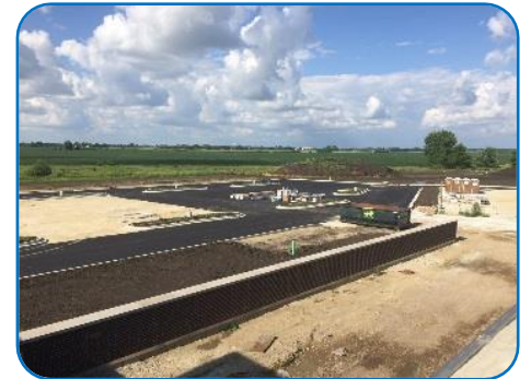
Employee Parking Lot Binder Coat
