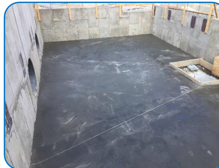
Freshly Poured Range Mechanical Unit Area – before the floor & roof
