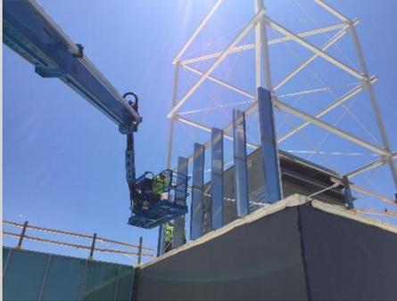
Metal panel bracing is being installed on the east side of the tower. These panels will enclose the entire tower, containing one mechanical unit and solar thermal technology. The solar thermal system will utilize the energy from the sun to heat a water/glycol mixture which is pumped through the floor piping producing radiant floor heating.
