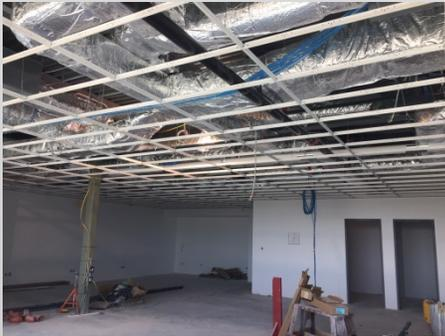
The ceiling grid in the Criminal Investigations area is complete, while the grid for the rest of the second floor is still in progress. Once all of the ceiling punch list items are complete, the ceiling tiles will be put in place.
