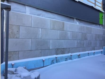
The stone wall along the training wing is complete. You will see the finished look once the metal panels are installed. The stone runs along the entire south wall of the training wing separated by glass enclosed "bump outs". These "bump outs" will act as break areas for staff during training days.
