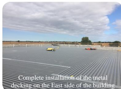
Complete installation of the metal decking on the East side of the building
