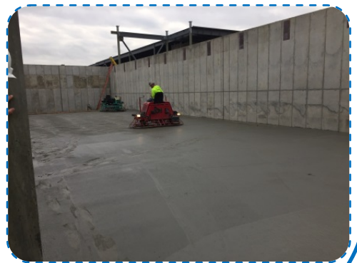
Range Floor - Poured
