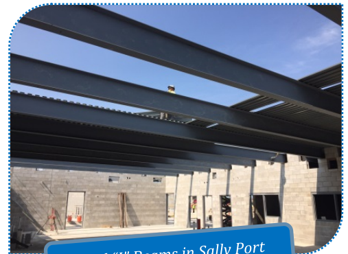
Steel "I" Beams in Sally Port
