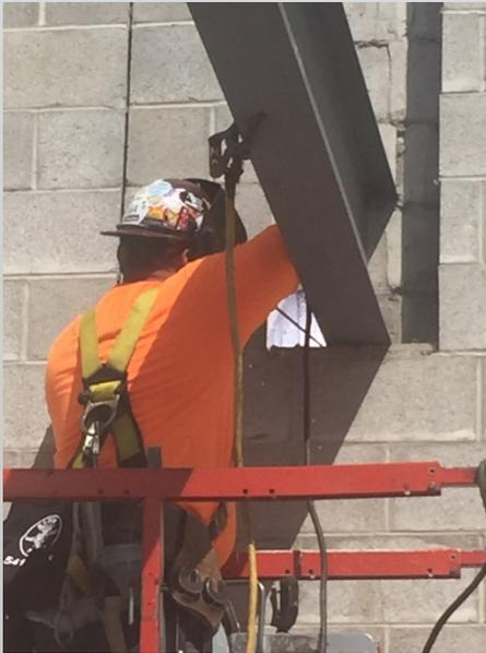
This "I" beam has been set into place and is being welded to the steel plate on the top of the brick. Crews will then fill in the beam pocket with additional block and grout.
