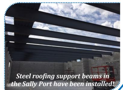
Steel roofing support beams in the Sally Port have been installed!
