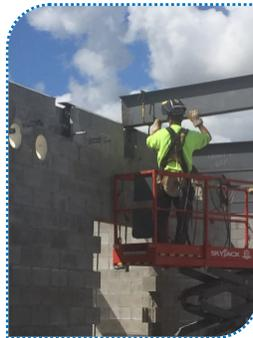
This steel "I" beam slides right into the masonry pocket and is welded into place. A perfect fit!
