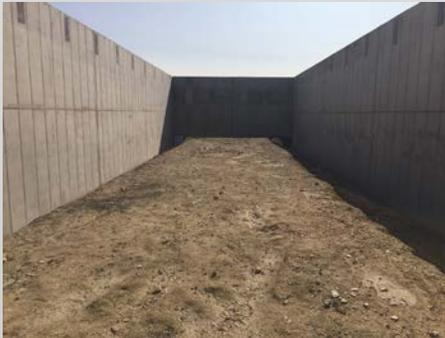
This picture shows the East end of the range (future location of the bullet trap). The walls are up with the steel and roofing to be added in a few weeks. The dirt that you see will be excavated in the coming weeks and the underground ventilation piping will be installed. Once that is done, the flooring will be poured. We can't wait to send rounds down range!
