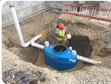
Crews installed the underground oil separator located in the Sally Port. The oil separator keeps any oil by-product from getting into the storm sewer.
