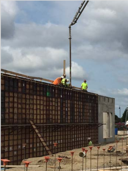
Construction of the North Range Walls!
