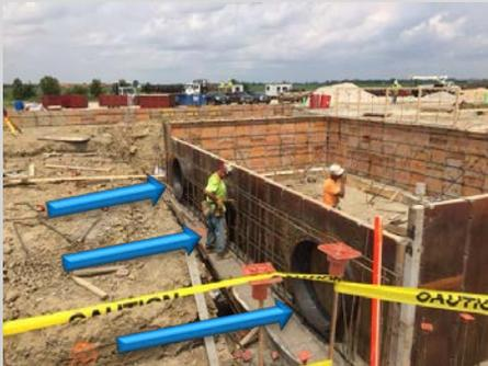
This is a picture of the training wing mechanical pit. The three future air handling pipes will be 3' in diameter running the length of the range under the floor! Wow!
