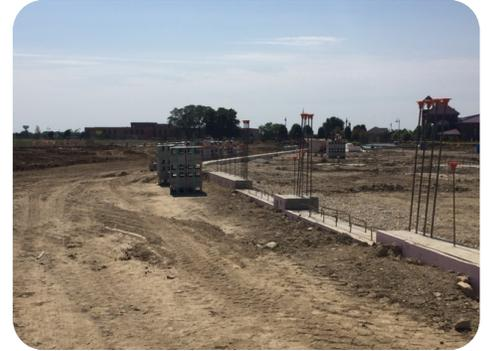
**The walls are going up!** Block has been delivered and work has begun on the Southeast garage walls. As expected, Masonry work will continue for the rest of this year and into next year. We have a long road ahead, but visible progress will be made each and every day!
