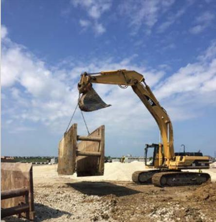
The trench box shown above was used to connect the Sanitary Sewer lines. To demonstrate how deep the lines run, the trench boxes were stacked on top of each other in the hole!
