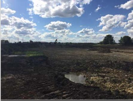
The final grade of the borrow pit is almost complete. There are a few areas that need additional shaping, but the overall size and depth of the pit is complete. S & K will be taking black dirt from the pile and spreading it out on the borrow pit to give it that clean, ready to plant look.
